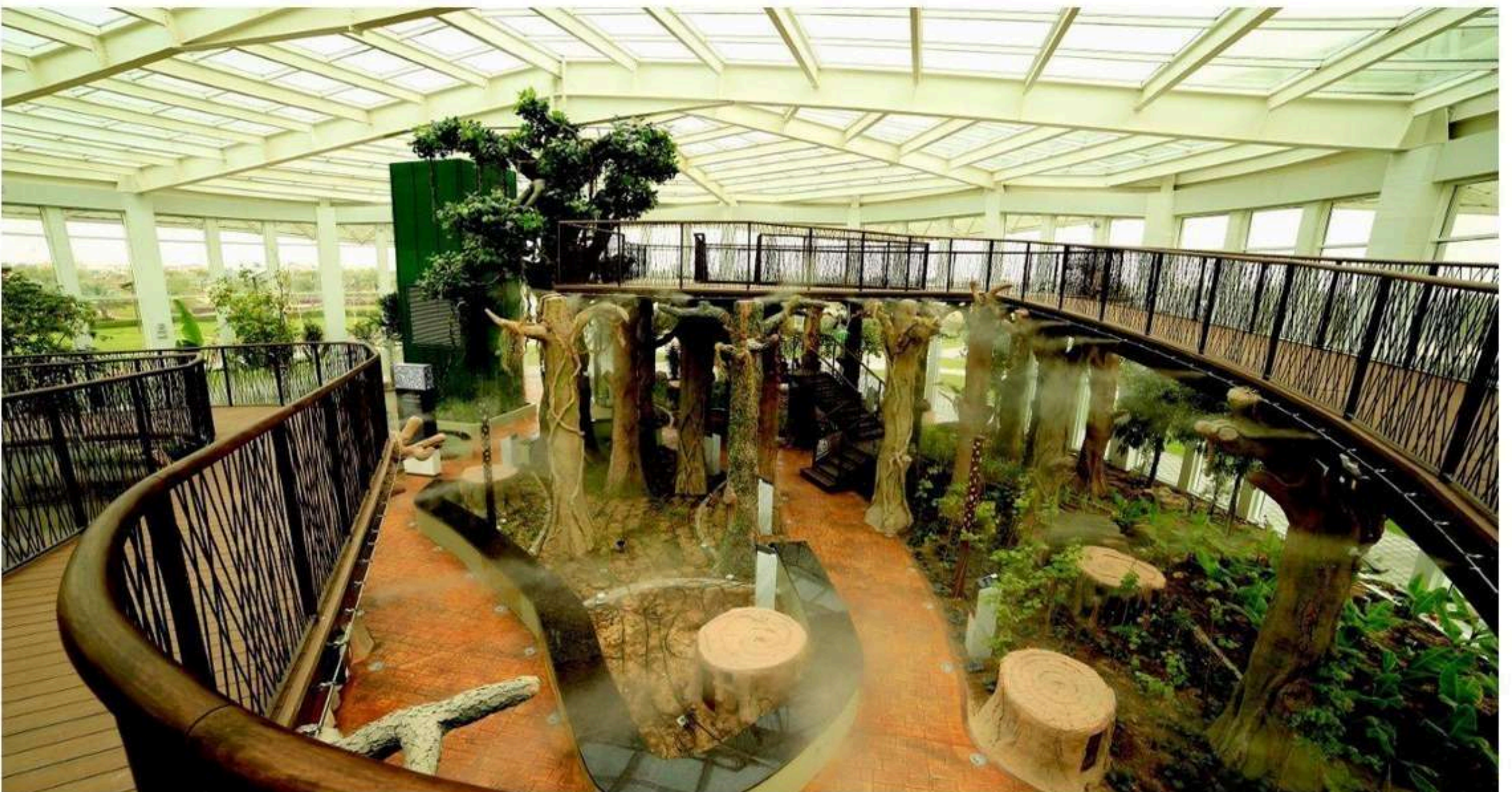
Stamped Concrete Work at Quran Park Kahwanej
