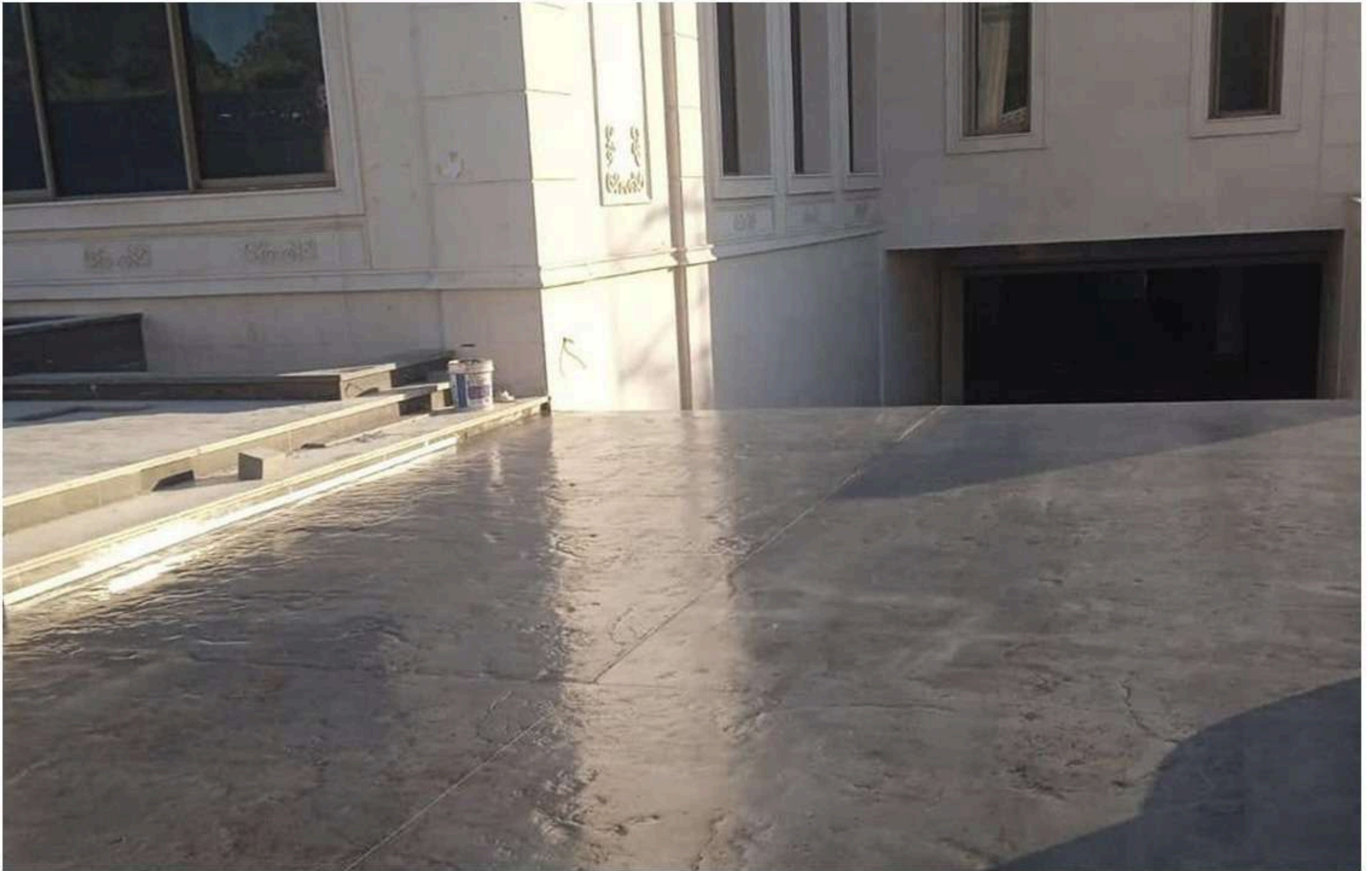
Stamped Concrete Work in Abu Dhabi
