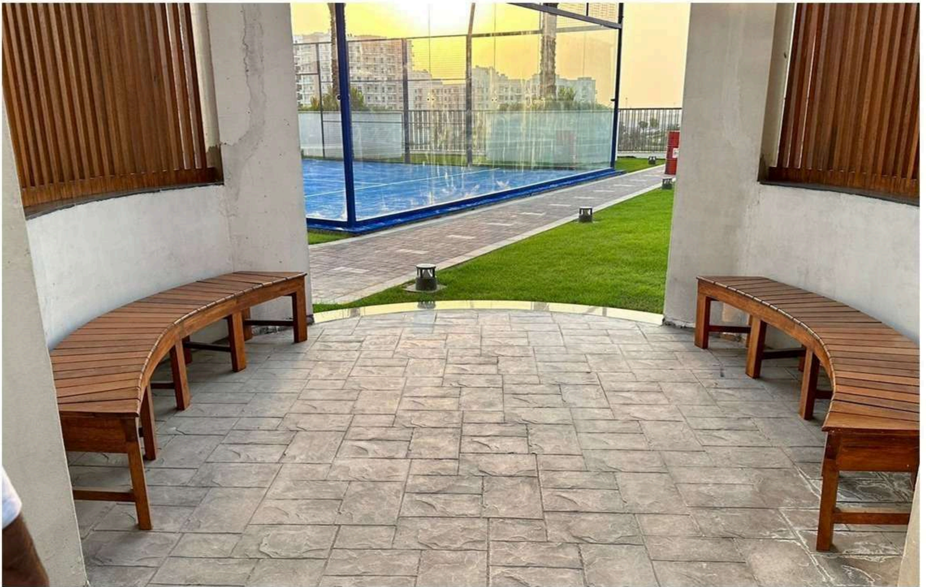
Stamped Concrete Work in Dubai
