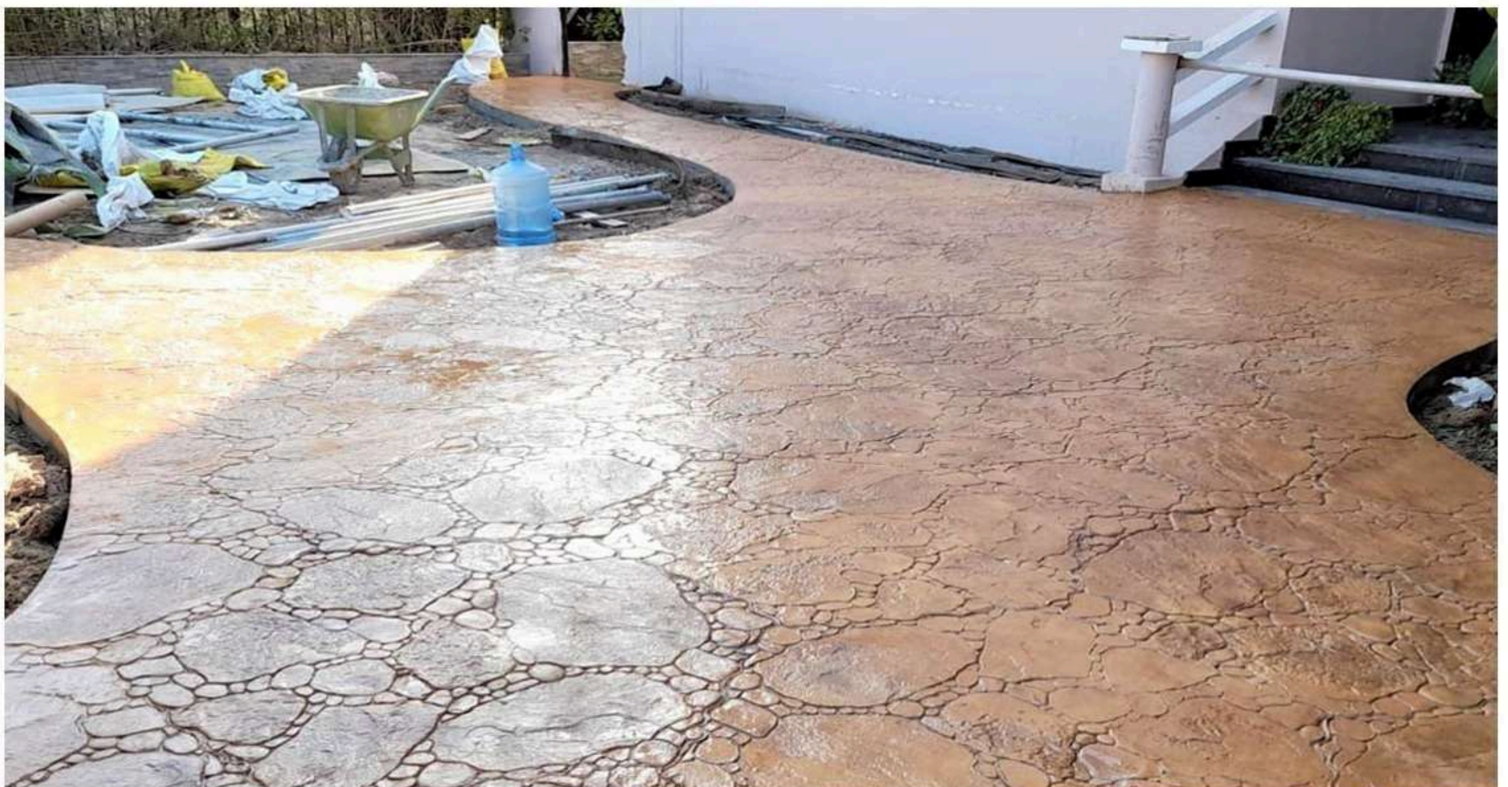
Stamped concrete work in The Villa, Dubai
