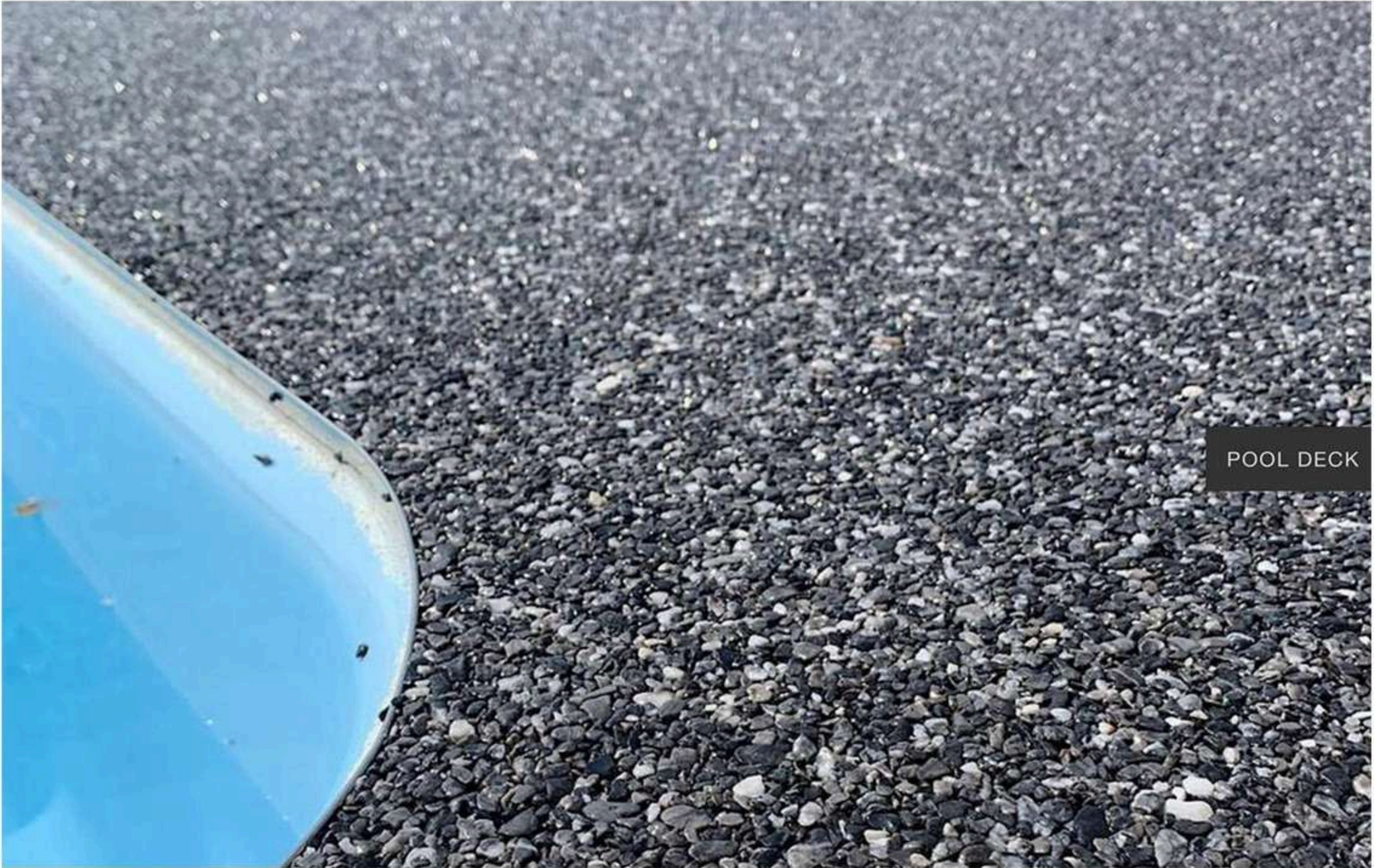
Pool Deck project at Dubai
