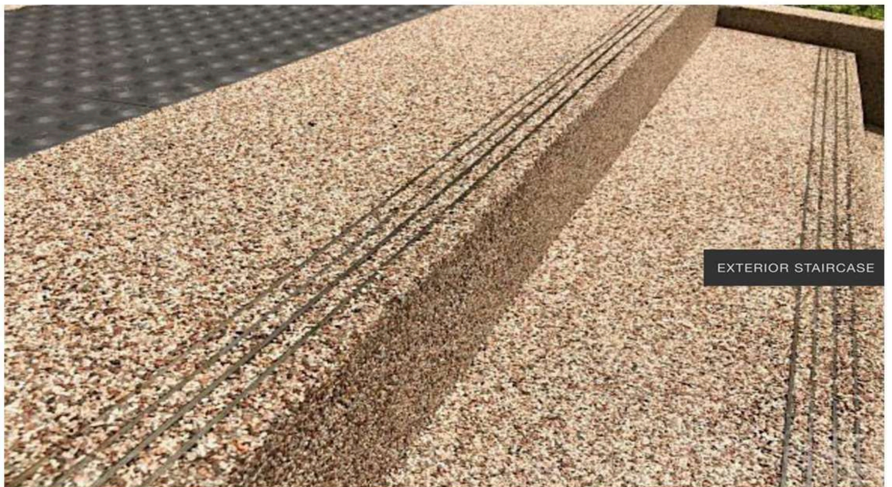
Exterior Staircase project at villa project
