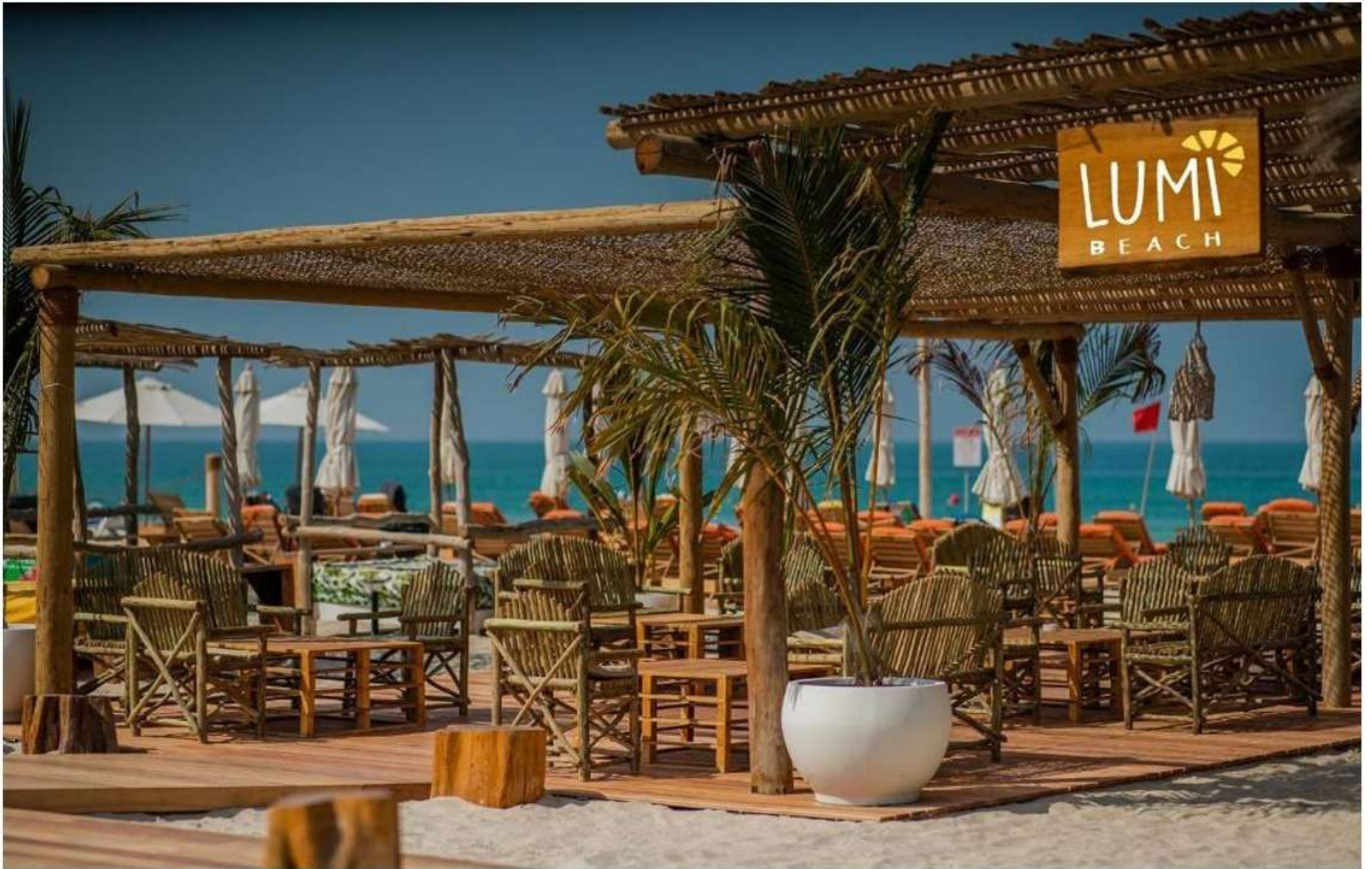
Render System Work at Lumi Beach
