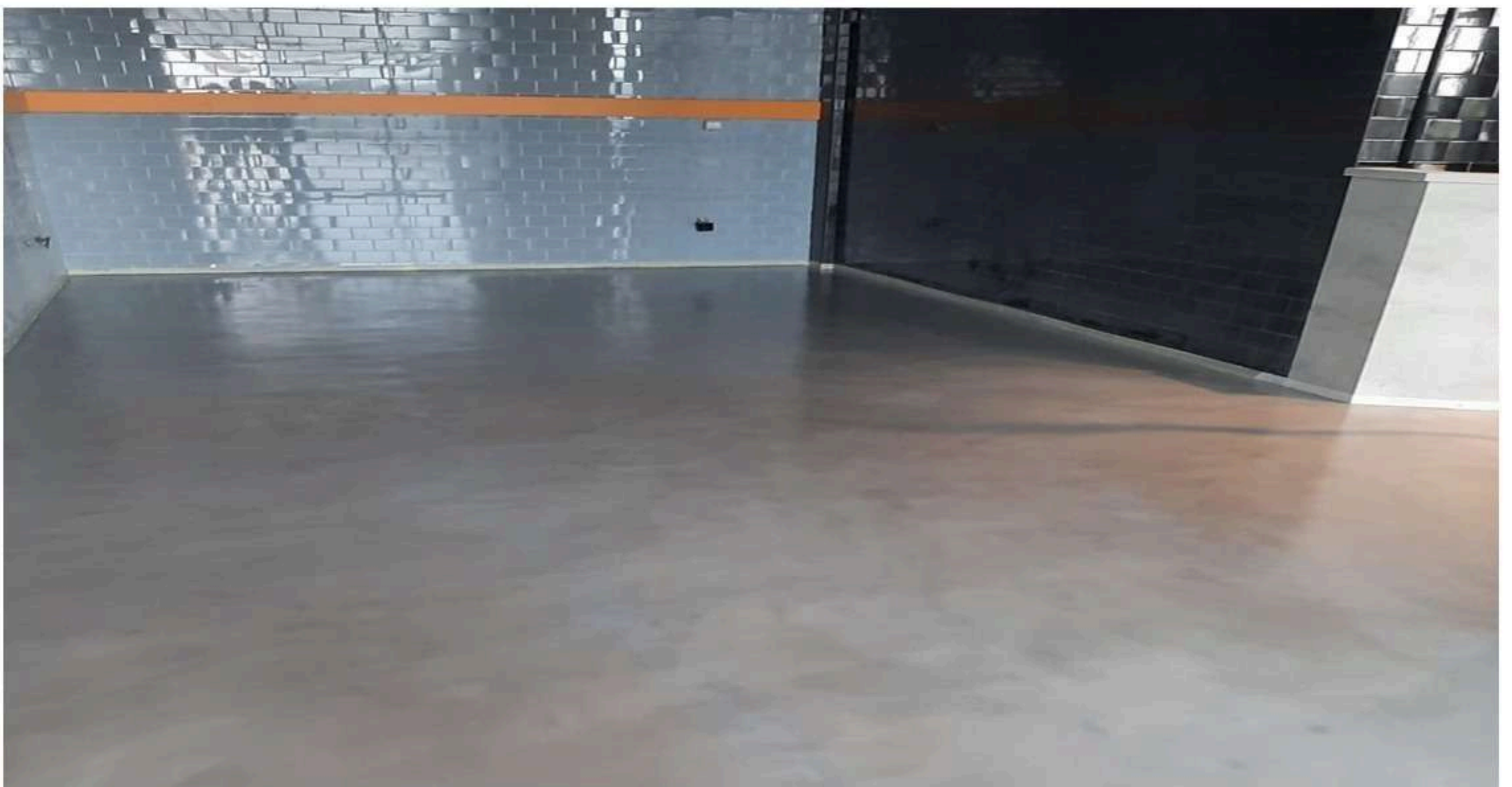
Microtopping Work at coffee shop in Khawanej
