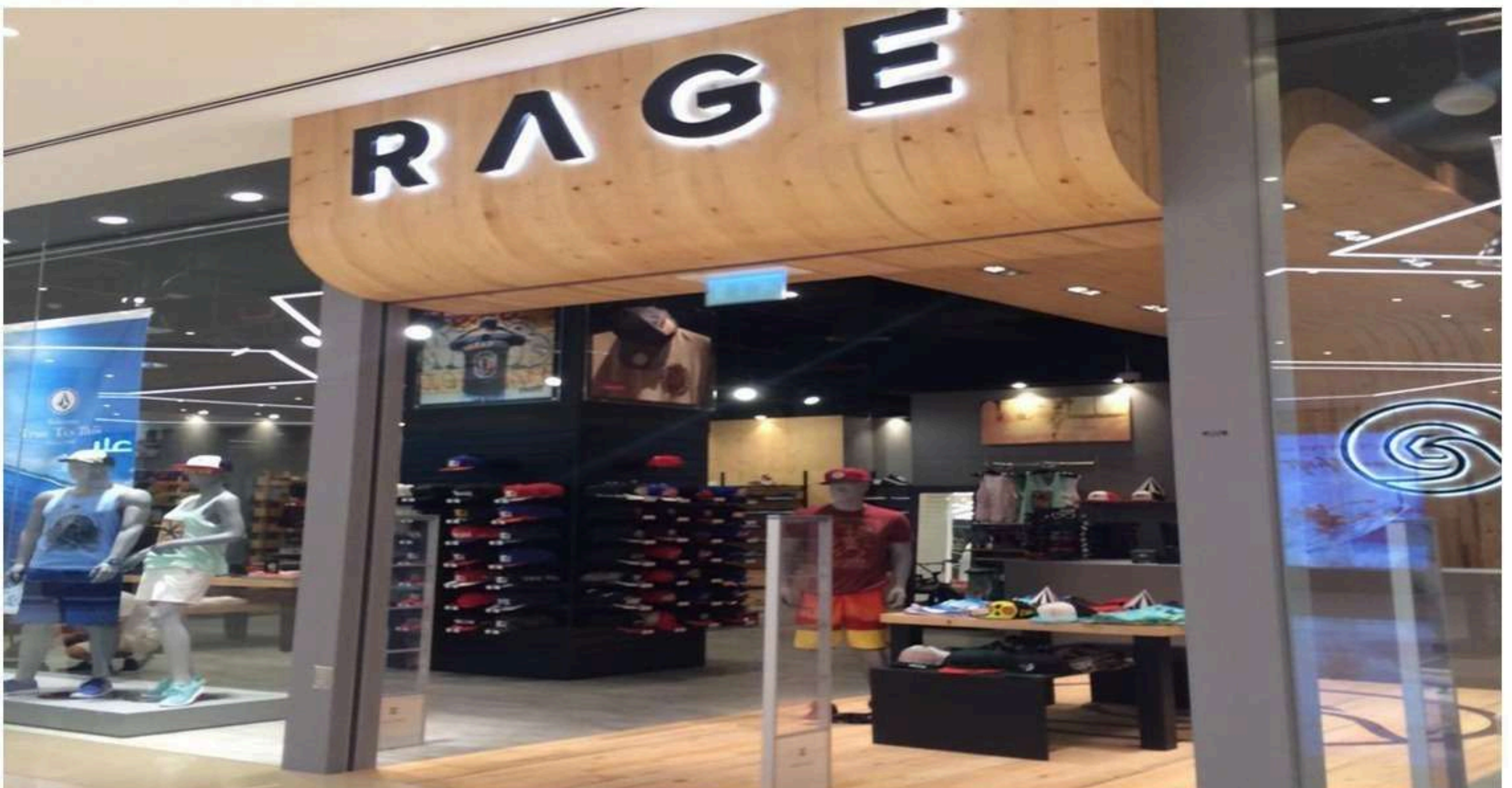
Microtopping Work at Rage Nakheel Mall
