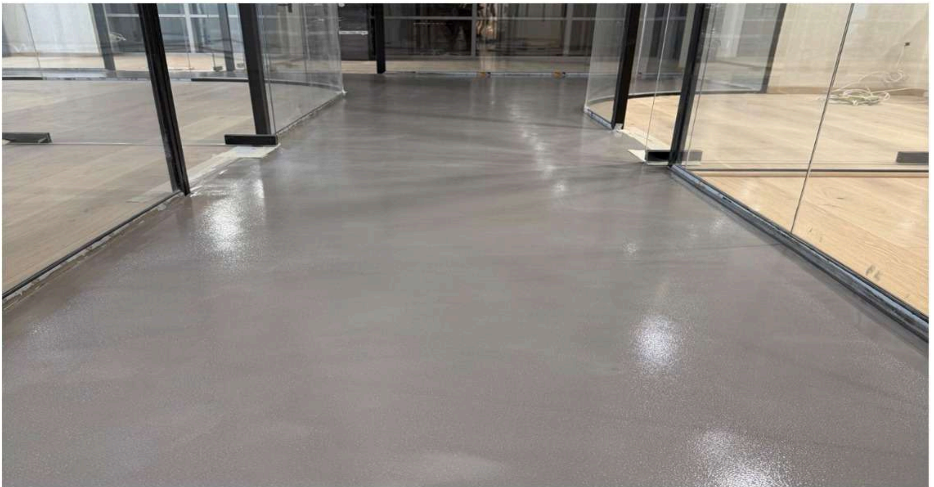
Microtopping Work at Sherina 3 Plaza
