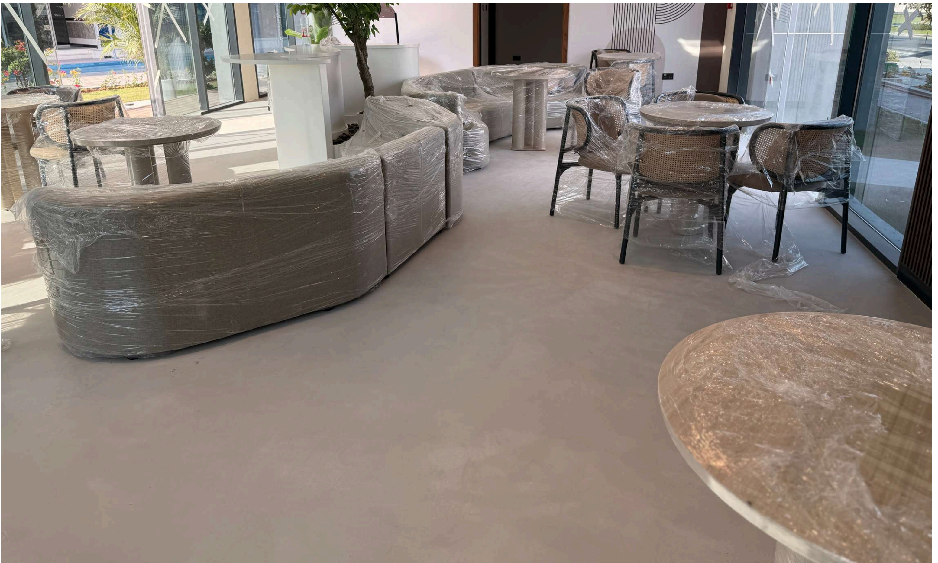
Microtopping Work in Ministry of Health, Muhaisnah
