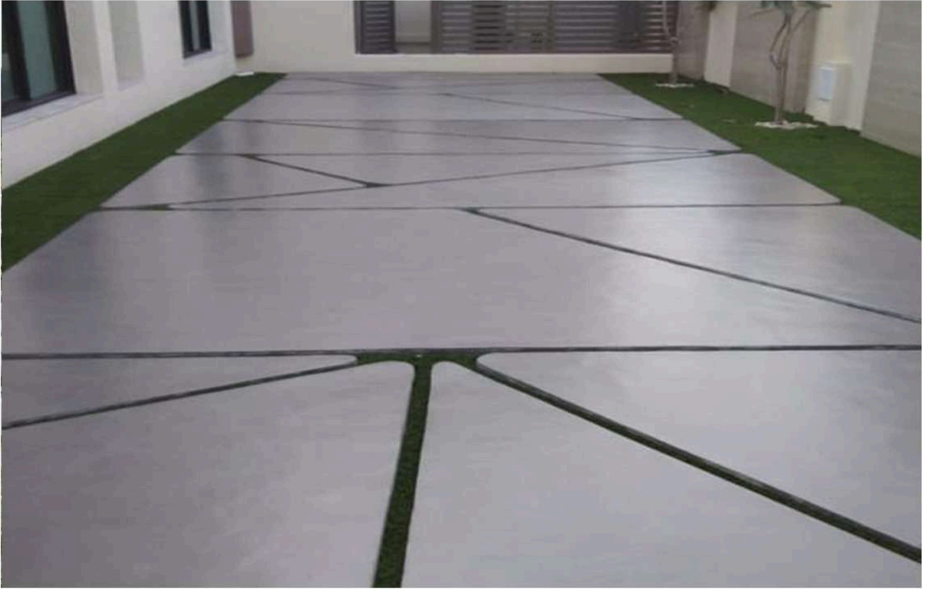
Microtopping Work at Dubai Sustainable City
