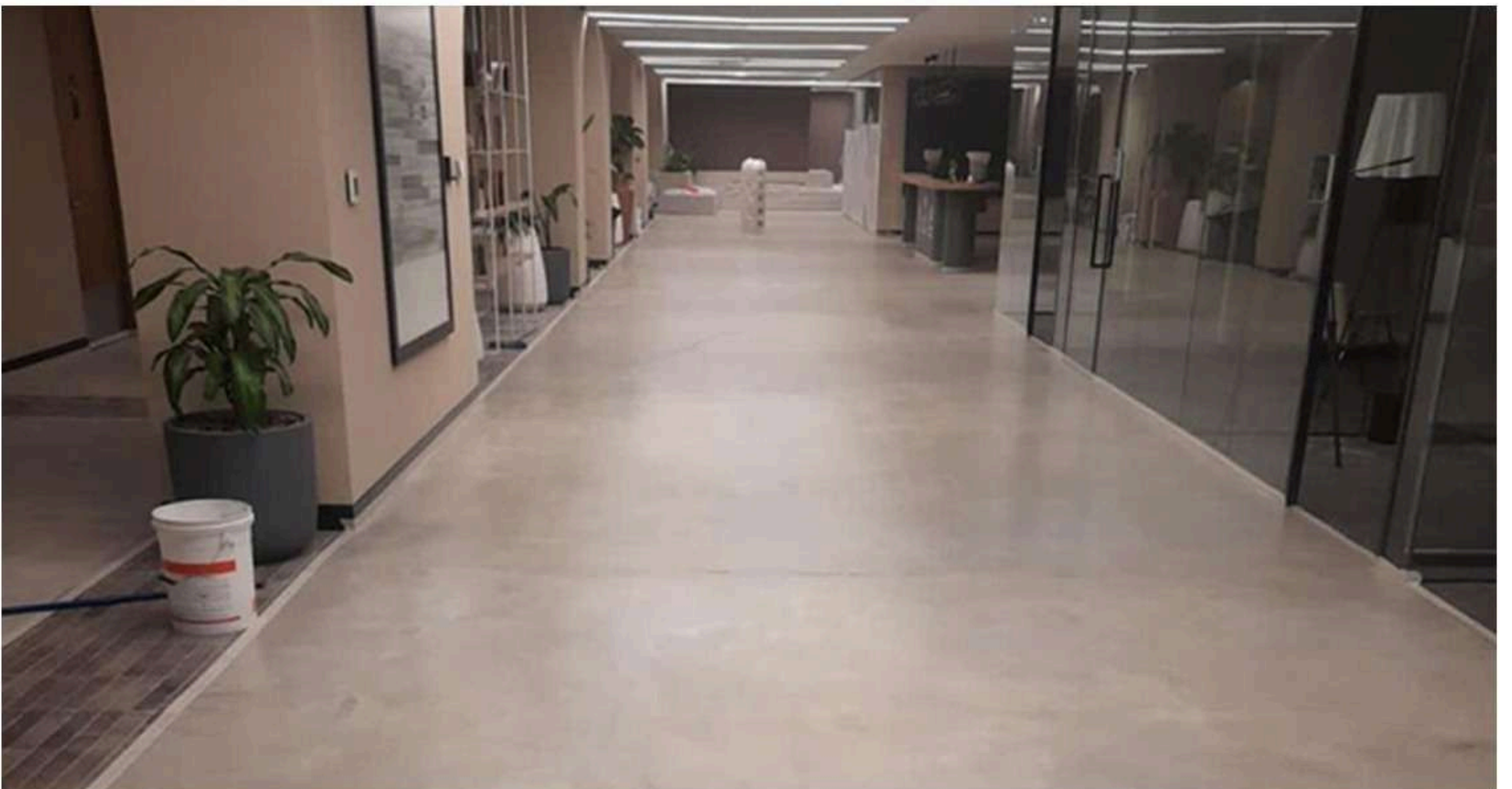
Microtopping Work in Dubai
