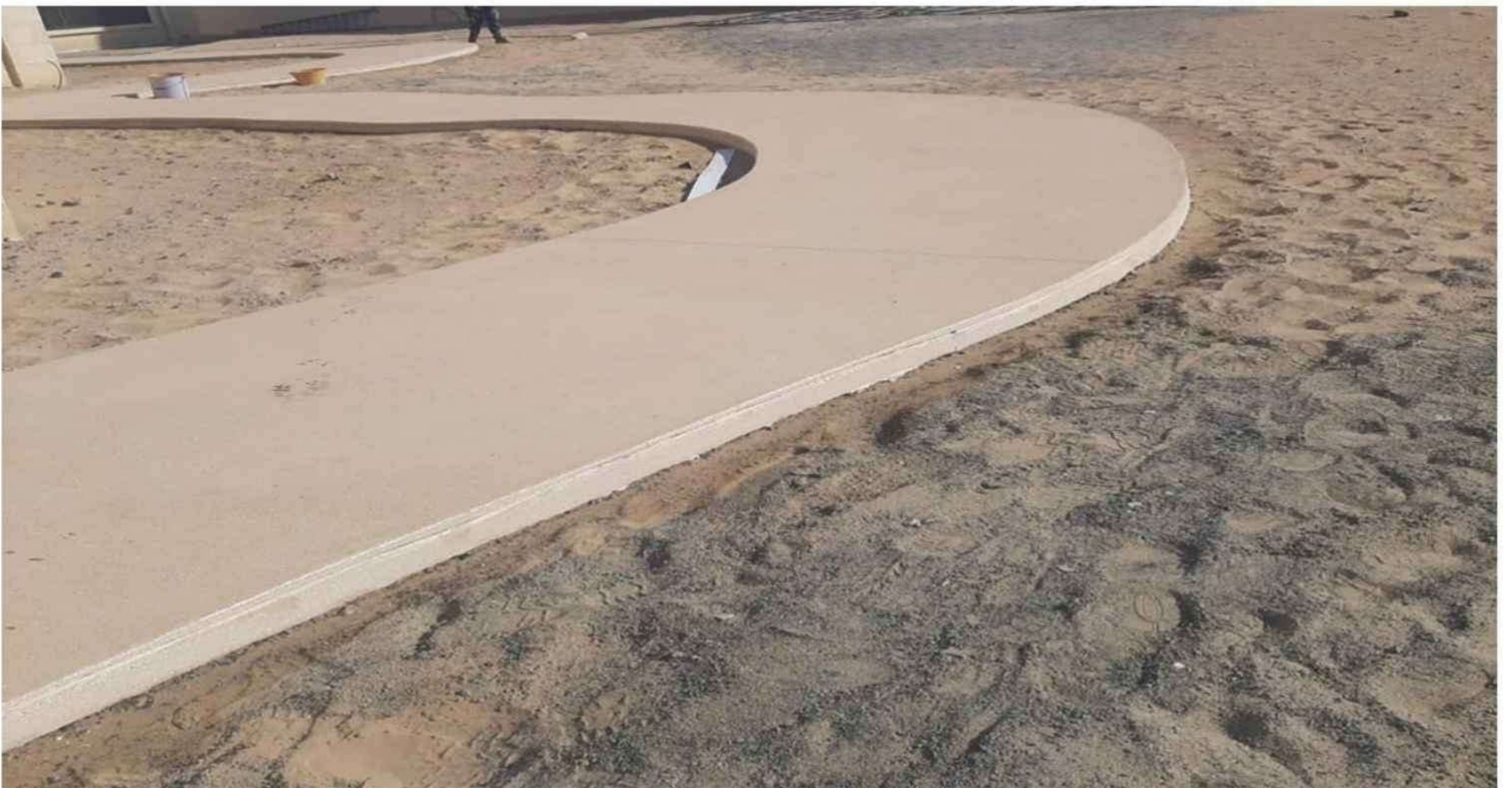
Exposed Aggregate Work at Private Villa
