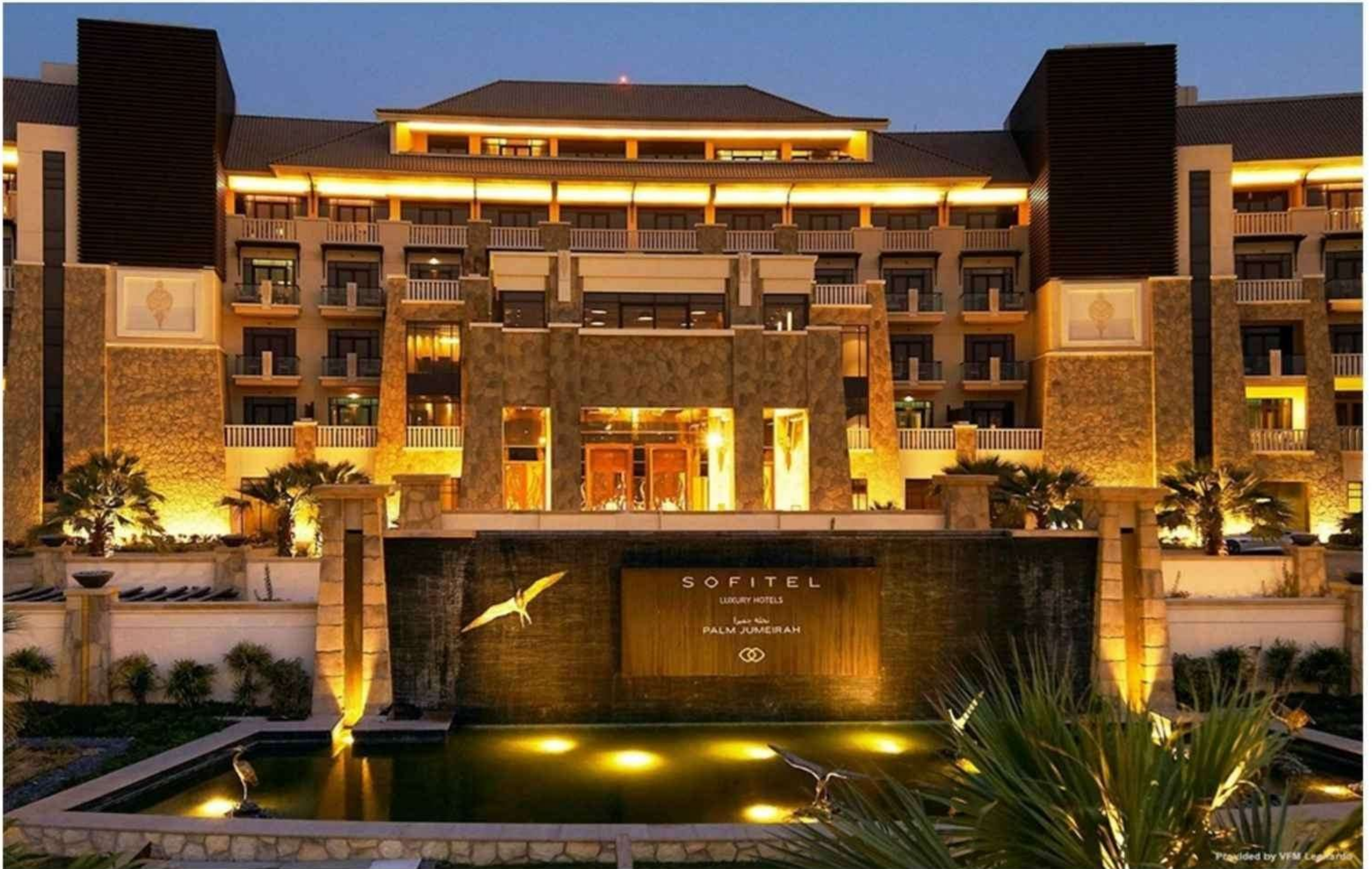
Exposed Aggregate Work at Sofitel The Palm
