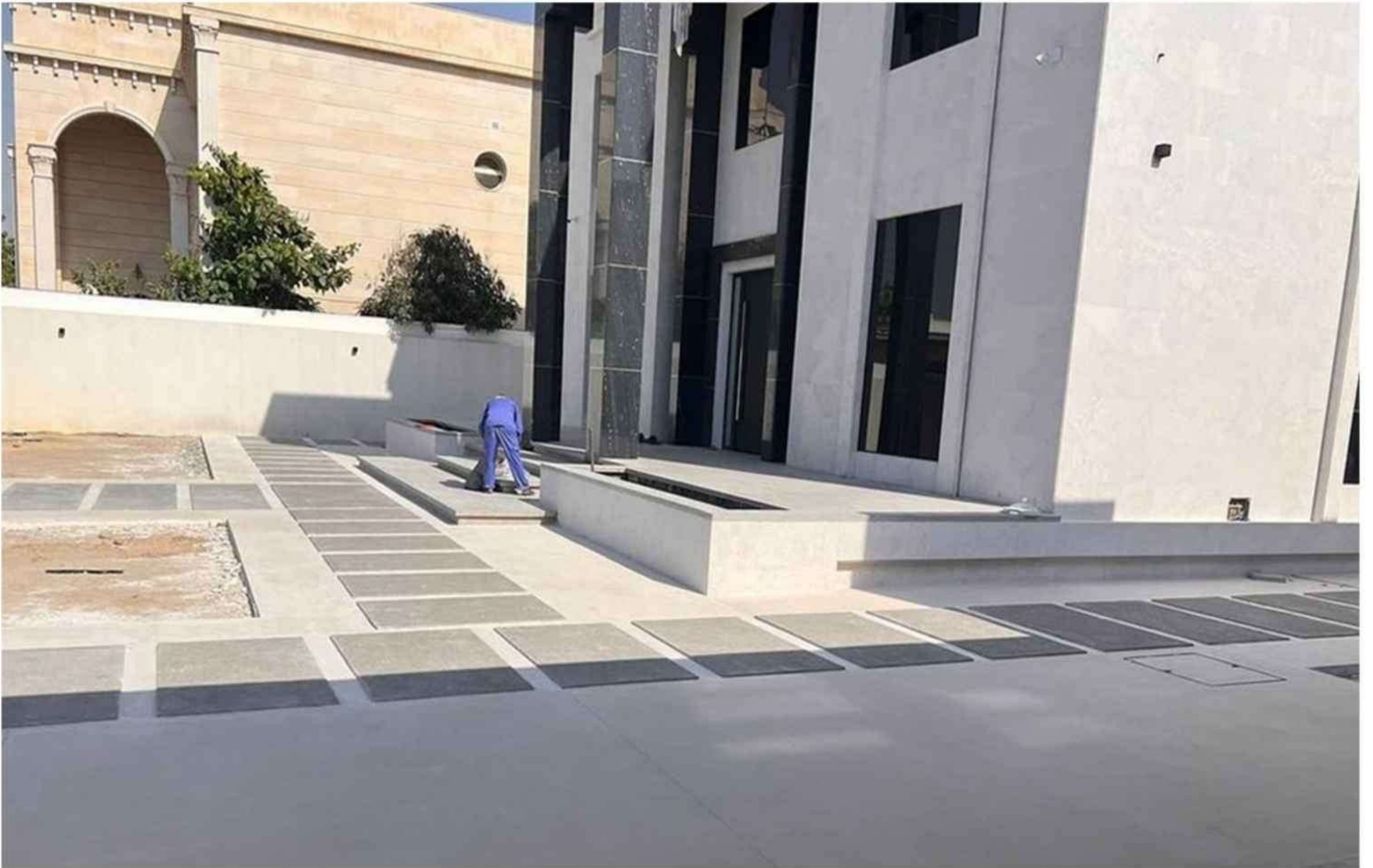
Exposed Aggregate Work at Al Mizher
