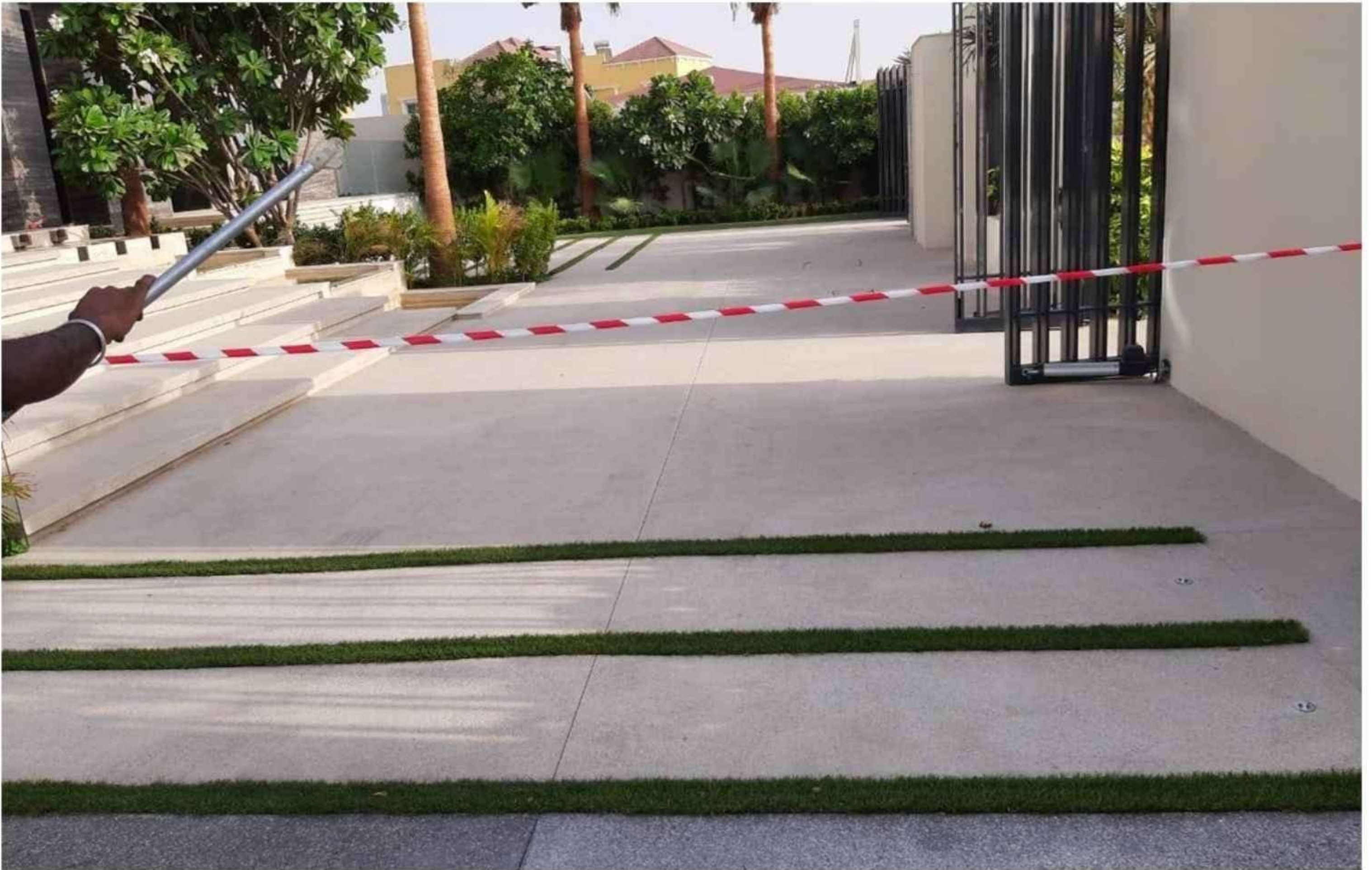
Exposed Aggregate Work at Nad Al Sheba
