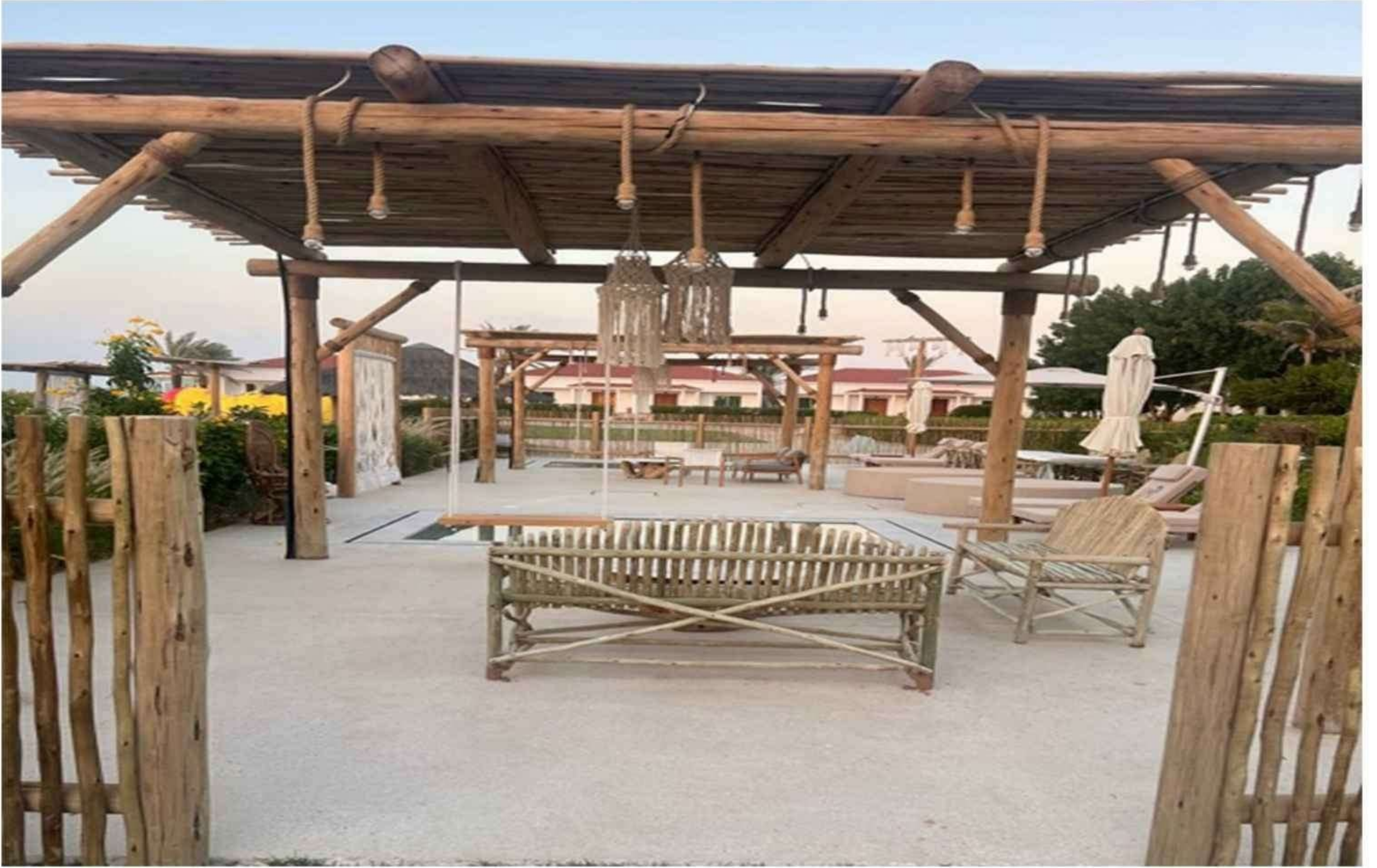
Exposed Aggregate Work at Lumi Beach
