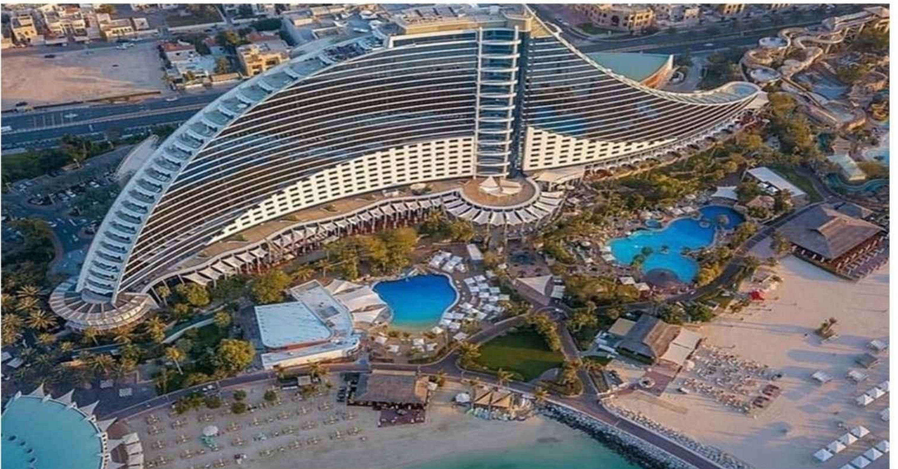
Exposed Aggregate Work at Jumeirah Beach Hotel
