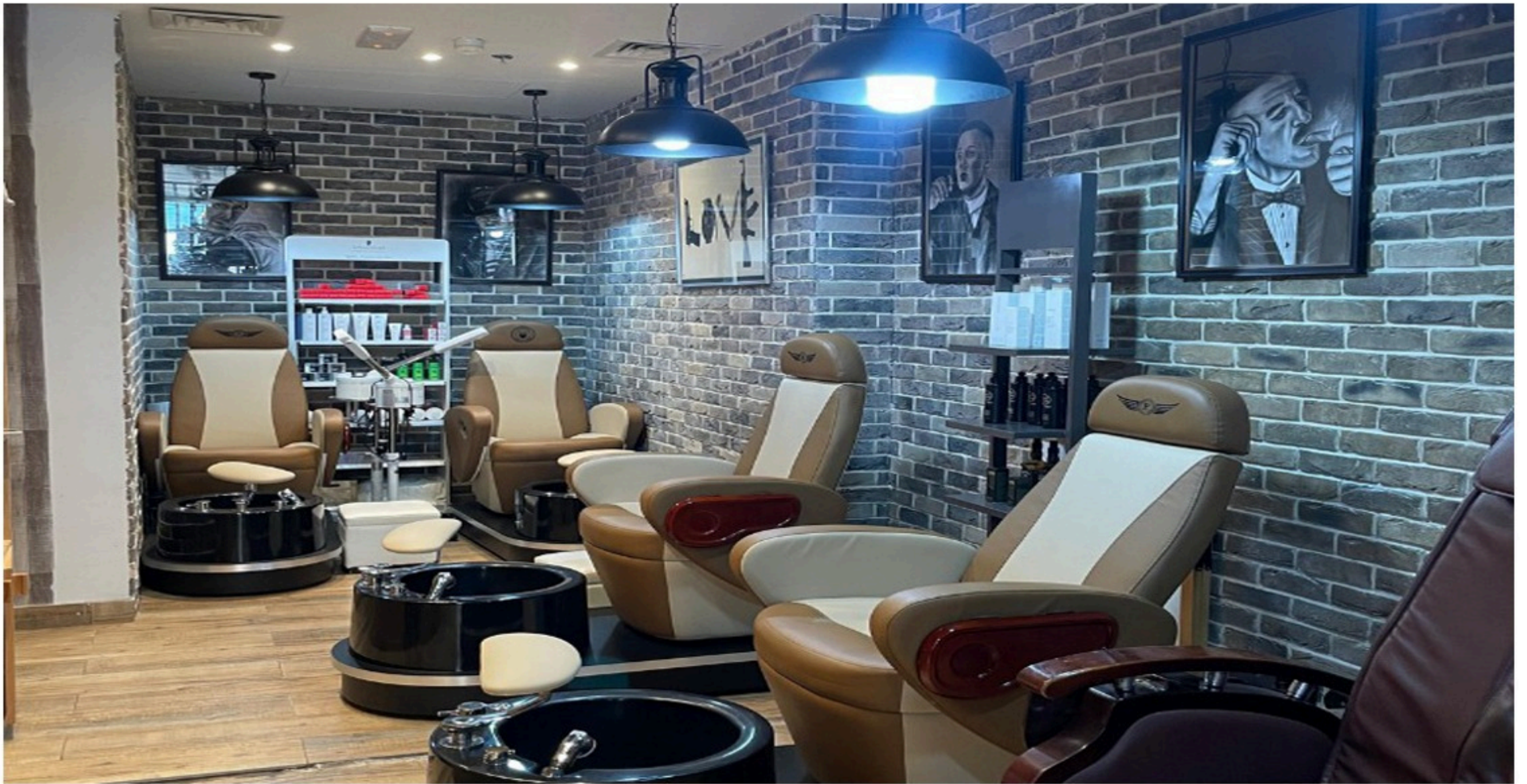
Brick Work at Peaky Blinder Barbershop, Five Jumeirah Hotel
