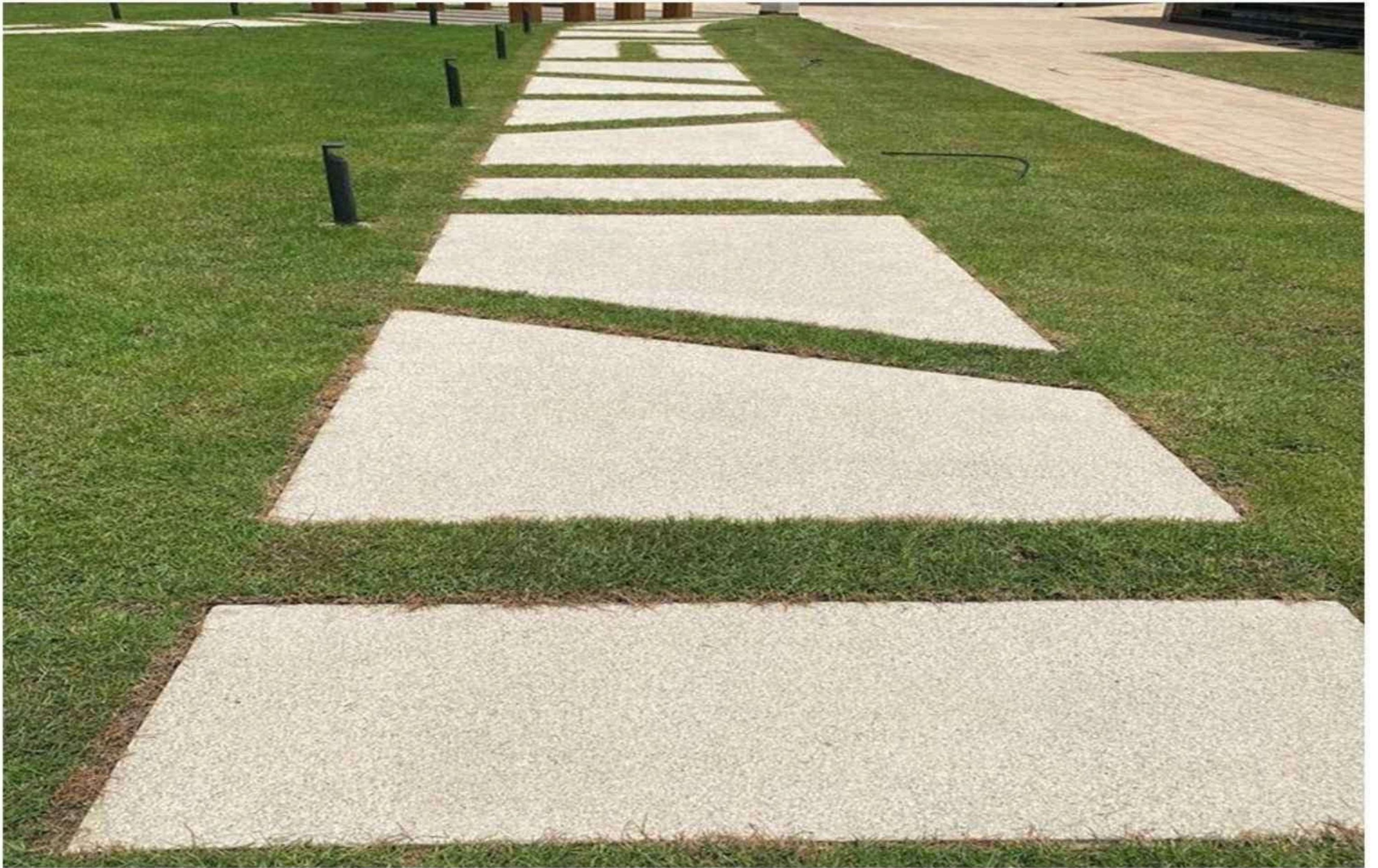
Exposed Aggregate Work at Nal Al Shiba
