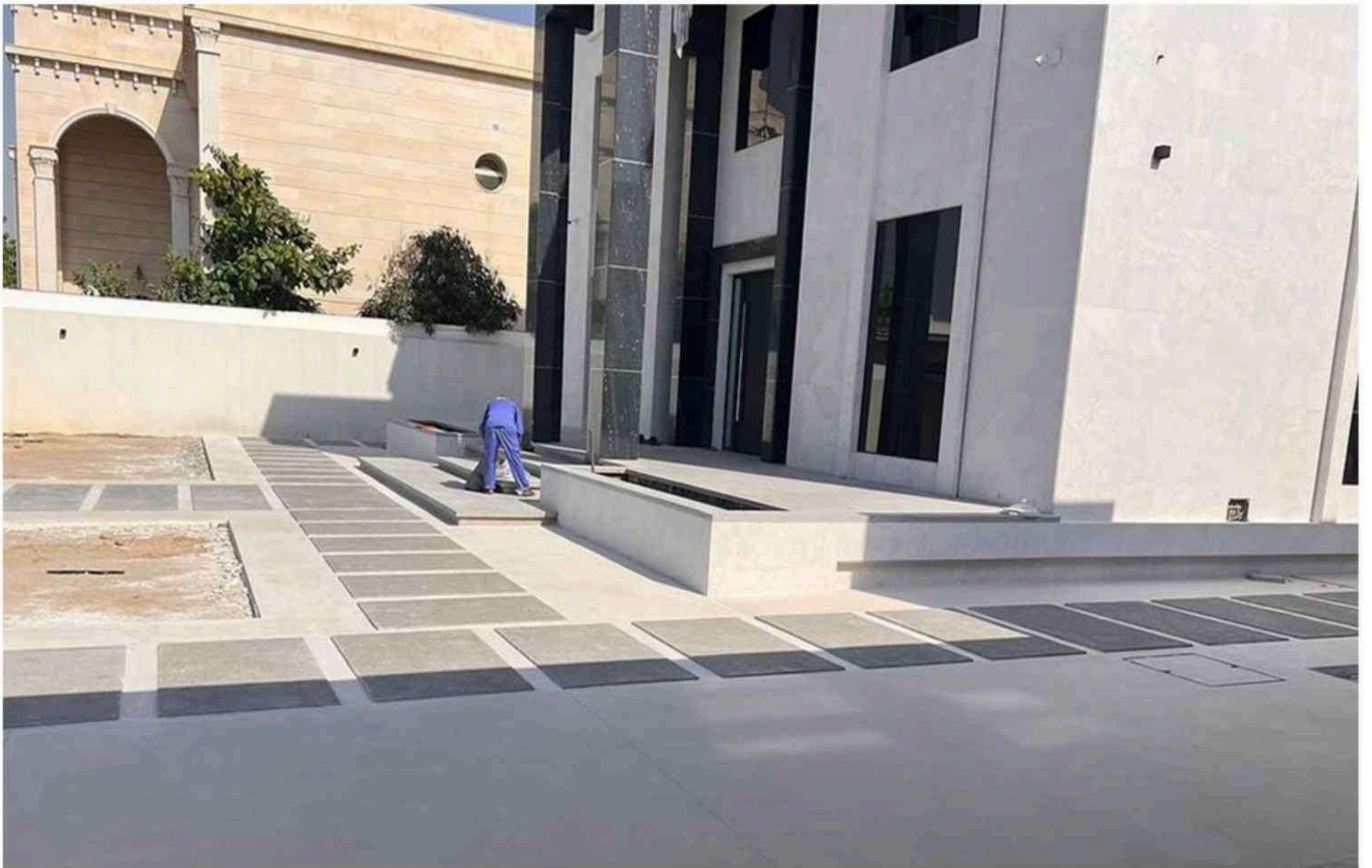
Exposed Aggregate Work at Al Mizher
